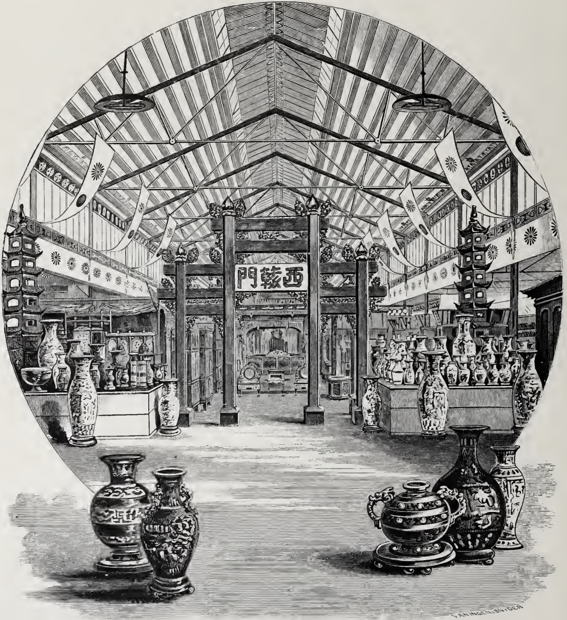
The Chinese Court—Main Building.
